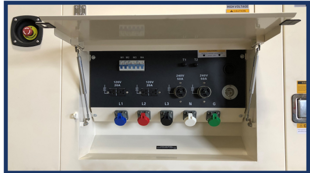
CUSTOMER CONNECTION PANEL
