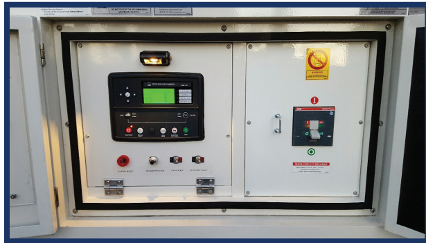
REAR CONTROL PANEL WITH MLCB
